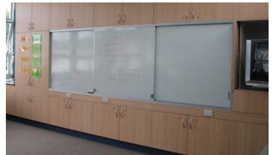
Henderson High School – Built-in storage units and large sliding whiteboards with storage behind them.
